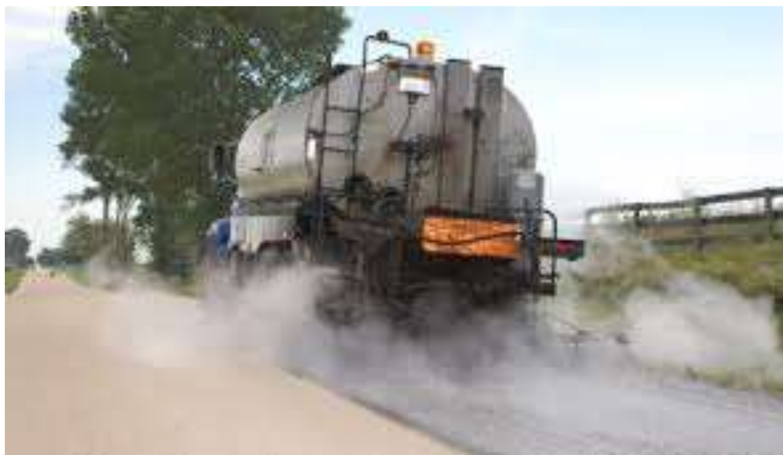
Figure D-1.5: Chip Seal Asphalt Operation
