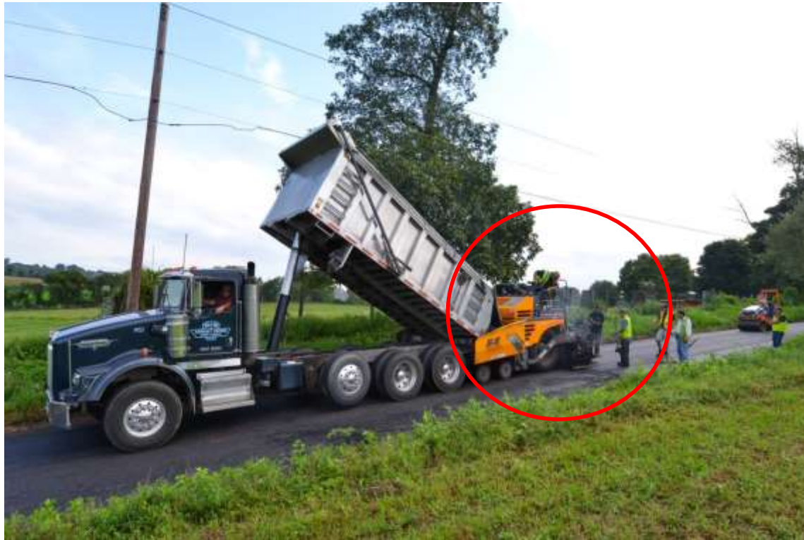
Figure D-1.2: Typical Jobsite Blue Smoke from the paver
