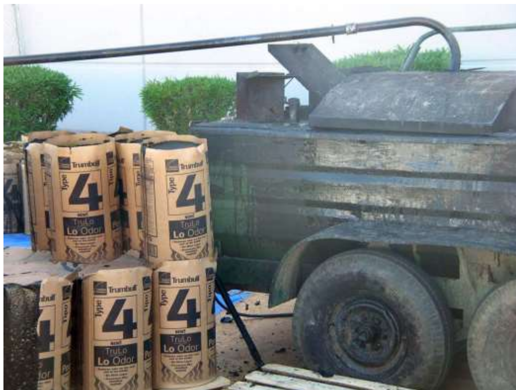
Figure IV-1: Roofing Asphalt Plugs, and Kettle
