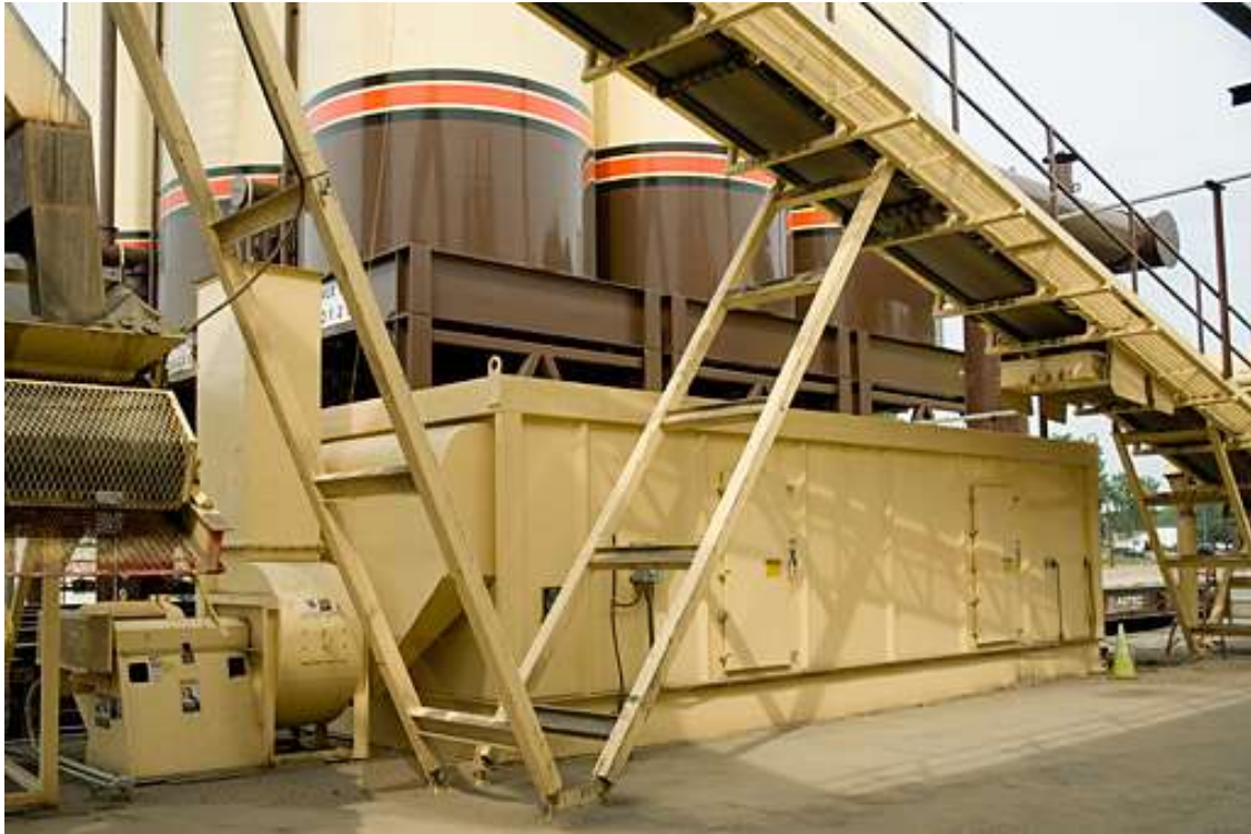
Figure D-1.4: Blue Smoke Abatement system with filters
