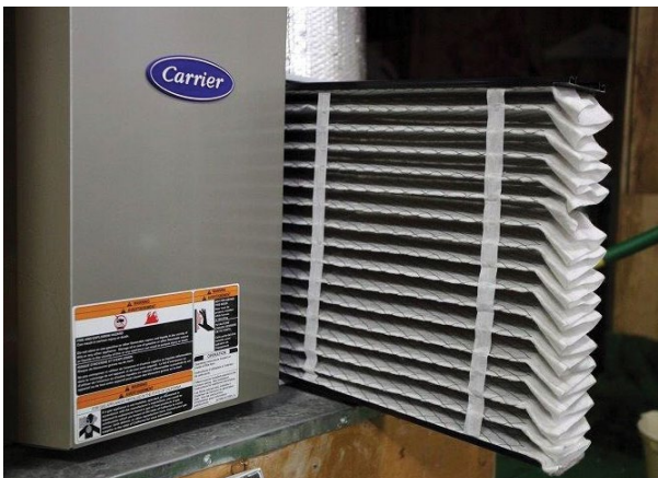
FORCED AIR FURNACE WITH HIGH EFFICIENCY FILTRATION (MERV 13 RATED)
