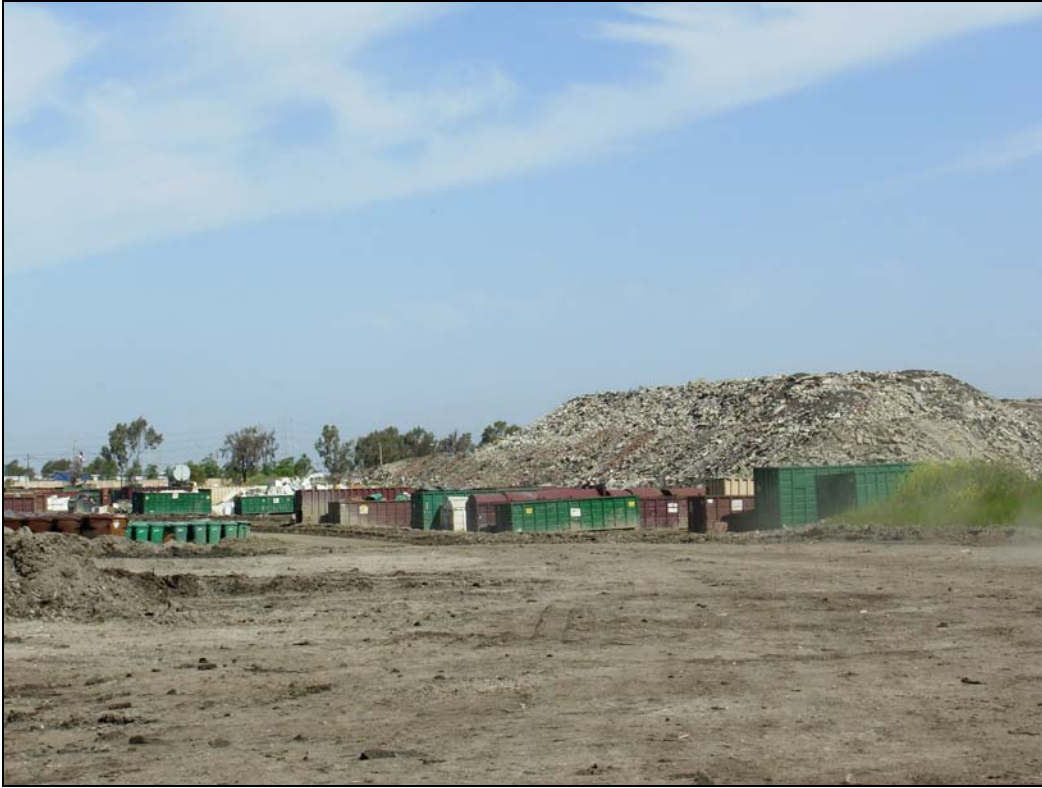
PHOTO 7. View of Resource Recovery Area looking north.
