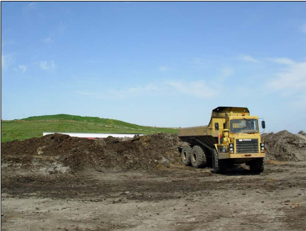
PHOTO 8. View of landfill from Resource Recovery Area, looking northwest.
