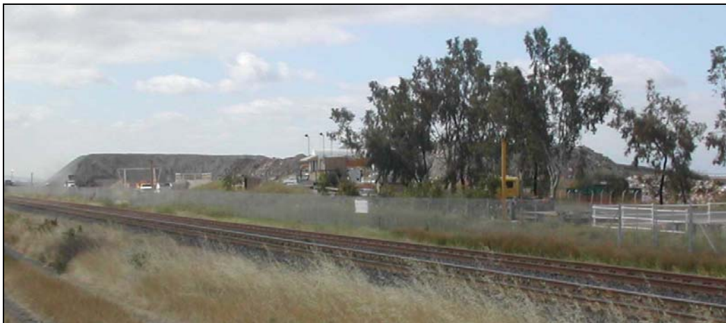
PHOTO 6. View of concrete recycling facility, looking southeast from Auto Mall Parkway near project entrance.
