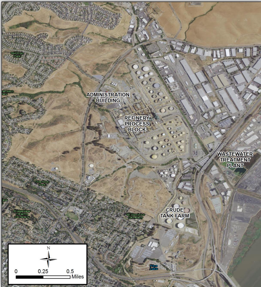
Figure 4. Layout of the Valero Benicia Refinery (Source of information: Valero Improvement Project Environmental Impact Report, June 2008).
