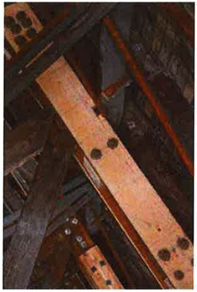
Chord sister repair installed prior to exoskeletons
