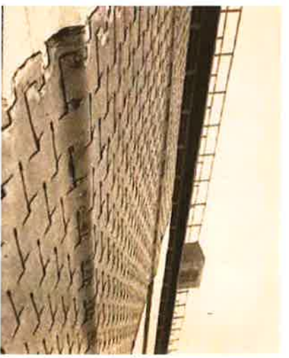
Asphalt shingles documented in 1954 -Seabees Historic Photos
