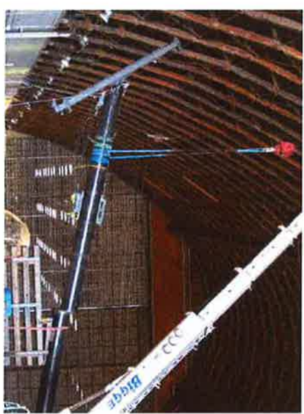
Hoisting of temporary shore segment
