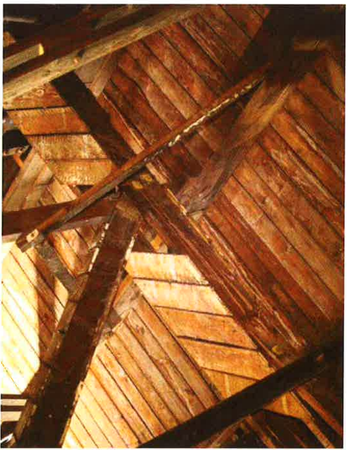
Typical vertical web member with added knee-braces
