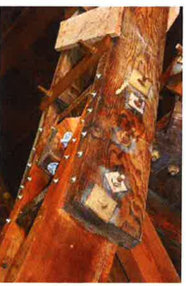
Preemptive screw and clamp strengthening on undamaged chord at node K
