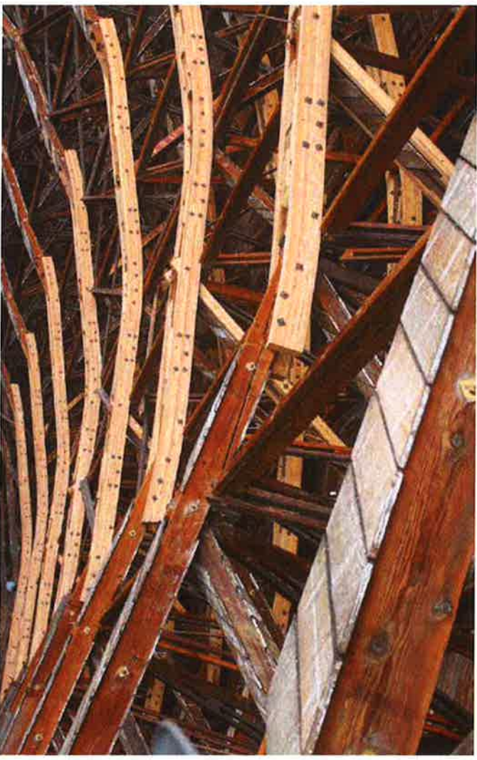
1993 glulam sister repairs to chord members in critical zone
