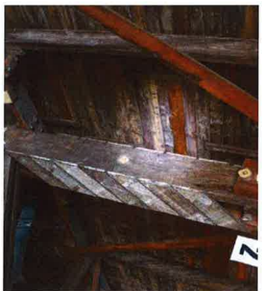
Typical chord member with battens
