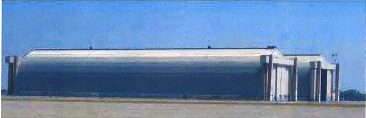
Figure 2. 2013 Hangar 2 (nearest hangar) and Hangar 3.
