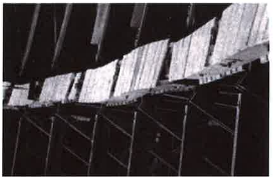
Buckled chords (left) and glulam strongback repairs (right) -“Restoration of Navy LTA (Lighter than air) Hangars”, Donal Neal, 1996
