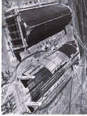
Hangars 2&3 under construction -US Navy Historic Photos
