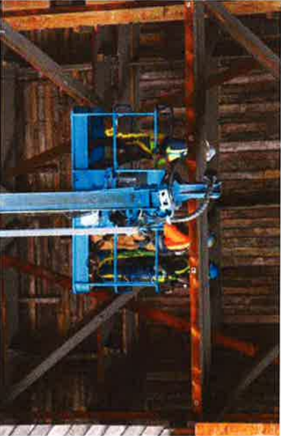
KPFF condition assessment crew
