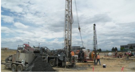
Installing vertical ground heat exchangers on a commercial geothermal system project
