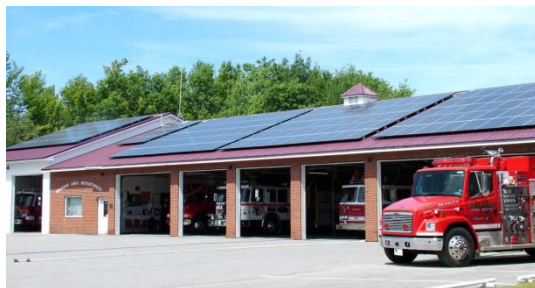
Resilient solar for critical facilities
