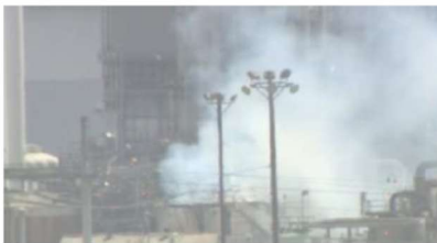
August 2016, Tesoro LA sulfur tank explosion.
