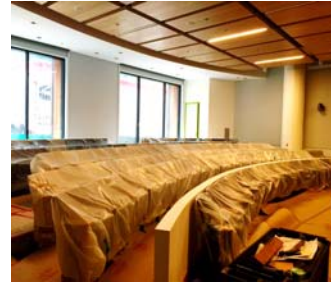
Board room seating installed
