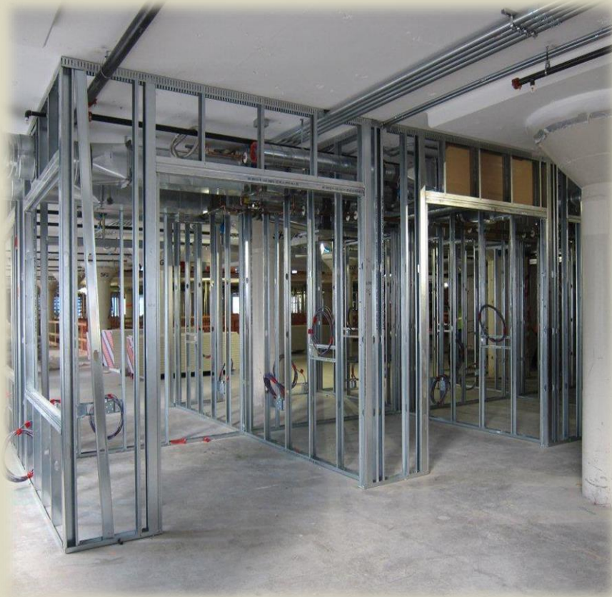
Figure 1: On Level 6 –Office Framing
