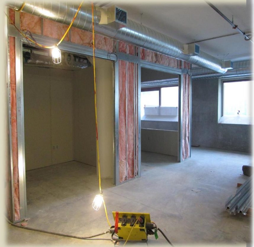
Figure 2: Offices being walled in on Level 6
