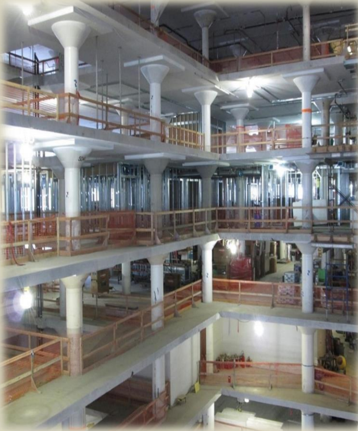
Figure 3: View across atrium of framing on Level 6
