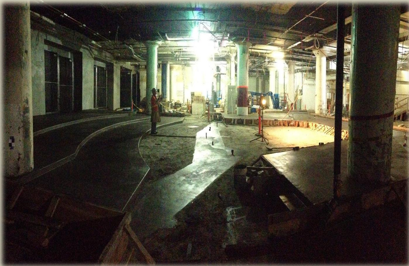
Figure 7: Concrete poured of board room seating and dias
