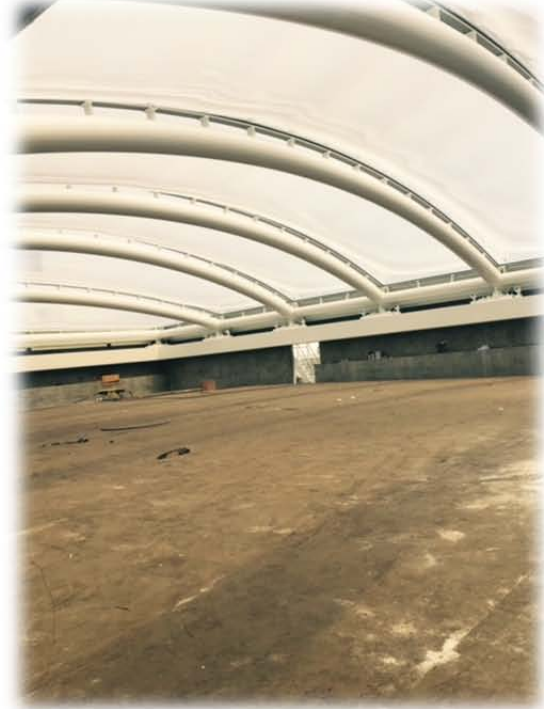
Figure 2: Atrium Skylight Glass in Place
