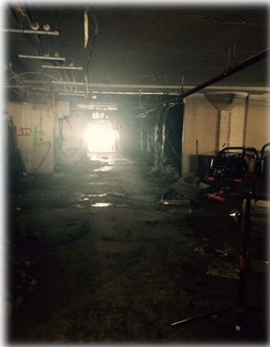
Figure 3: Demolition on Level 8
