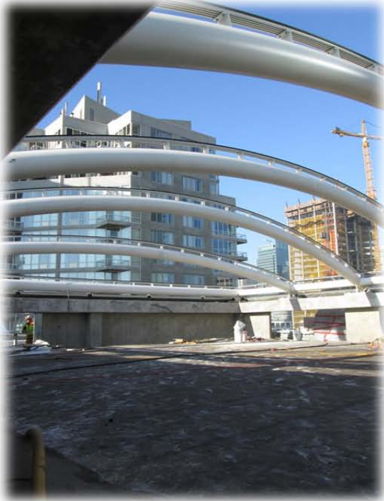
Figure 1: Atrium Skylight Support
