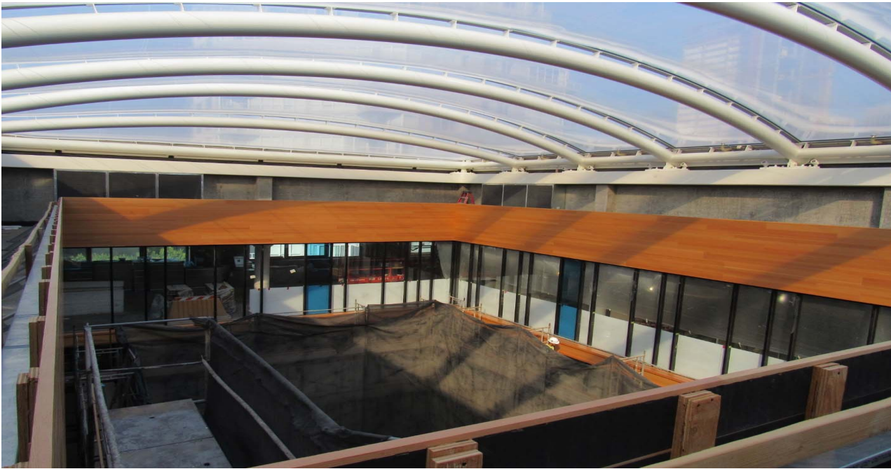
Figure 6: View from roof of atrium skylight – installation of wood framing and atrium glass enclosure
