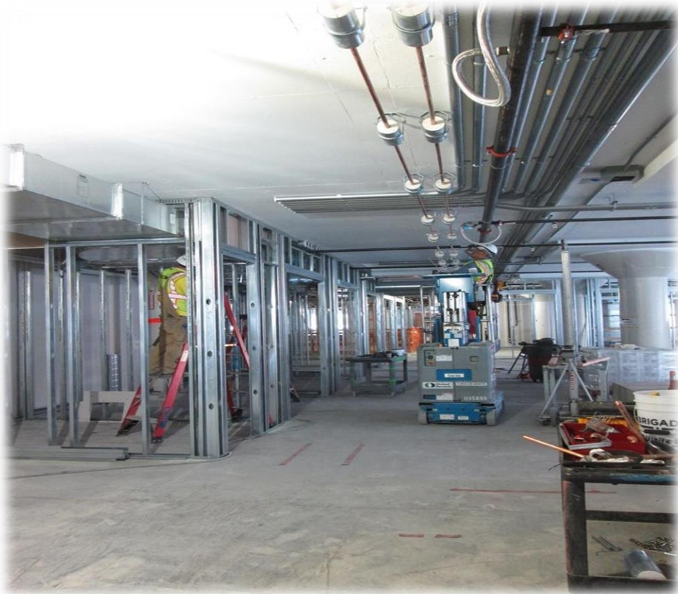
Figure 1: On Level 6 - Installation of office framing, utilities and plumbing overhead.
