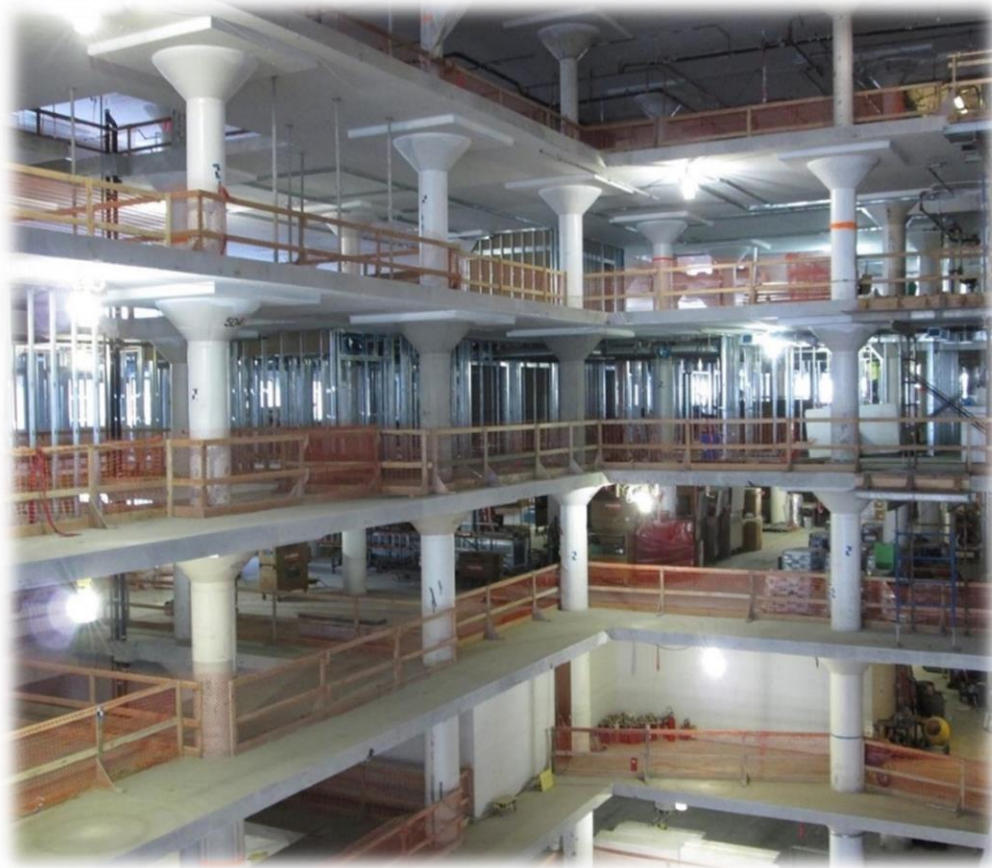
Figure 3: View across atrium of framing on Level 6
