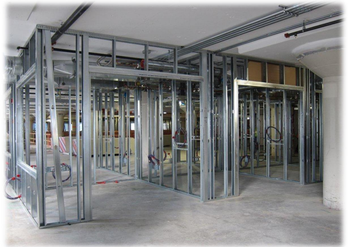
Figure 2: Office framing on Level 6
