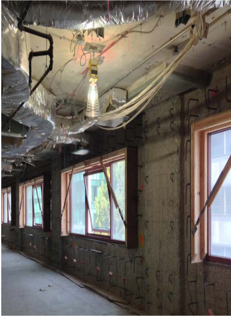
Rebar dowels installed on the perimeter walls. Concrete will be shot against the walls to seismically strengthen the building.
