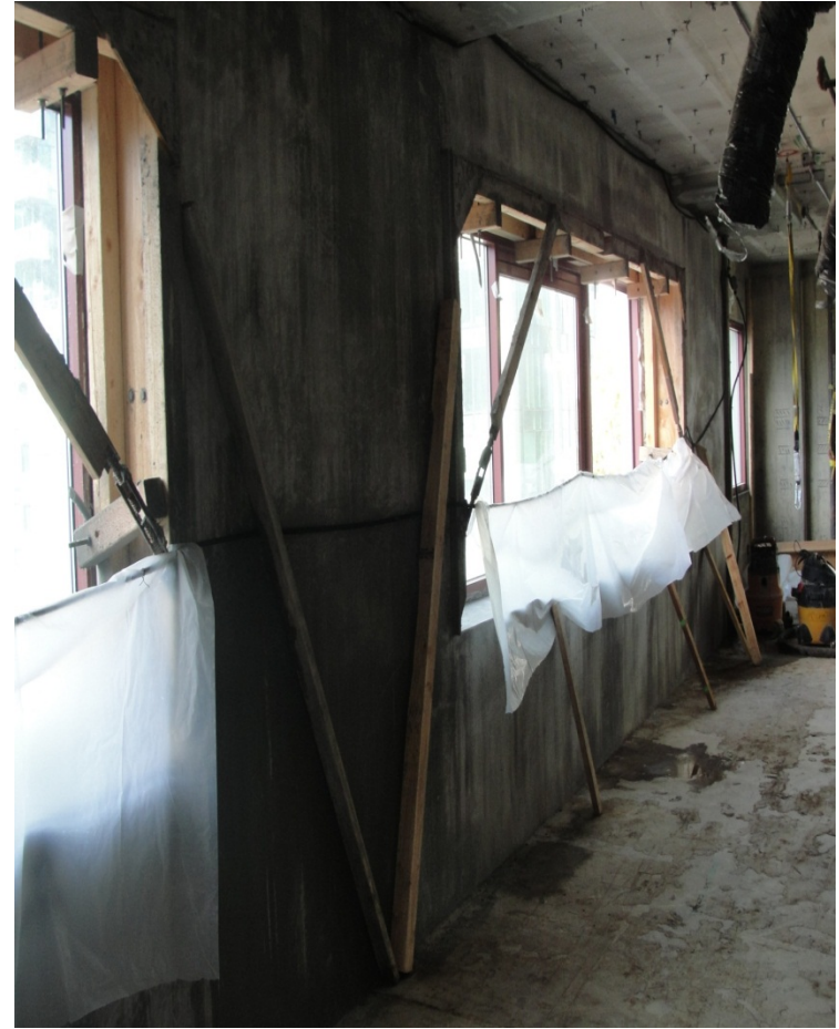
November - Shotcrete seismic retrofit work
