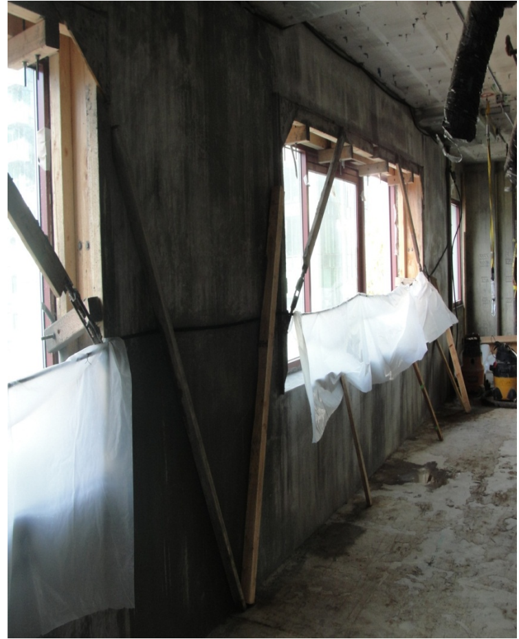
November - Shotcrete seismic retrofit work
