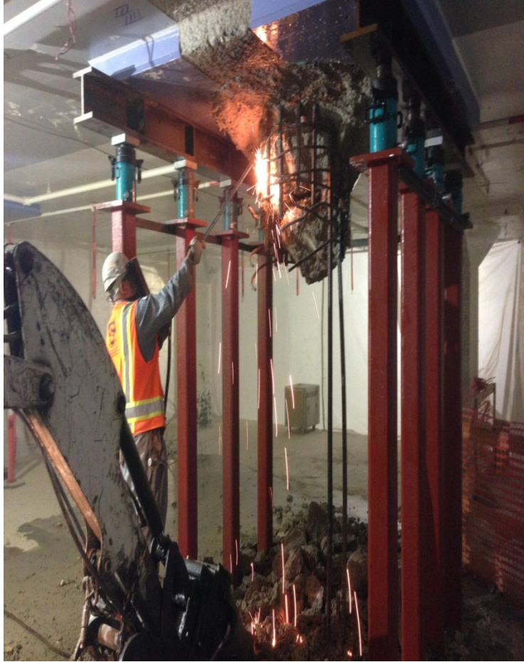
Removal of column above Multi-Purpose Room.
