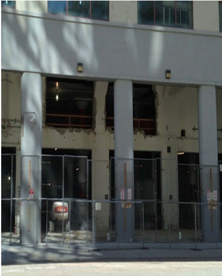
Beale Street entry: current condition.
