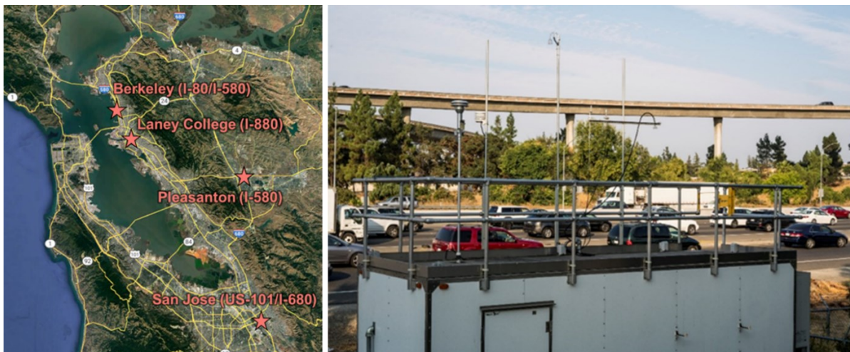
Figure 13. Locations of the Air District's near-road air monitoring sites (left) and photo of the San Jose-Knox St. near-road air monitoring site along the US-101/I-680 interchange (right).
