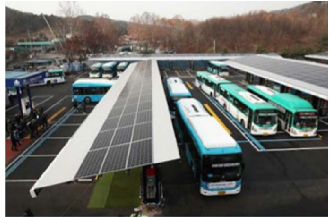
Above: Electric charging infrastructure; source: WestCAT Update and Overview
