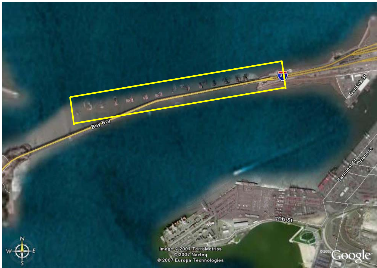
Figure 7. Assumed area for construction emissions from the Bay Bridge project.
